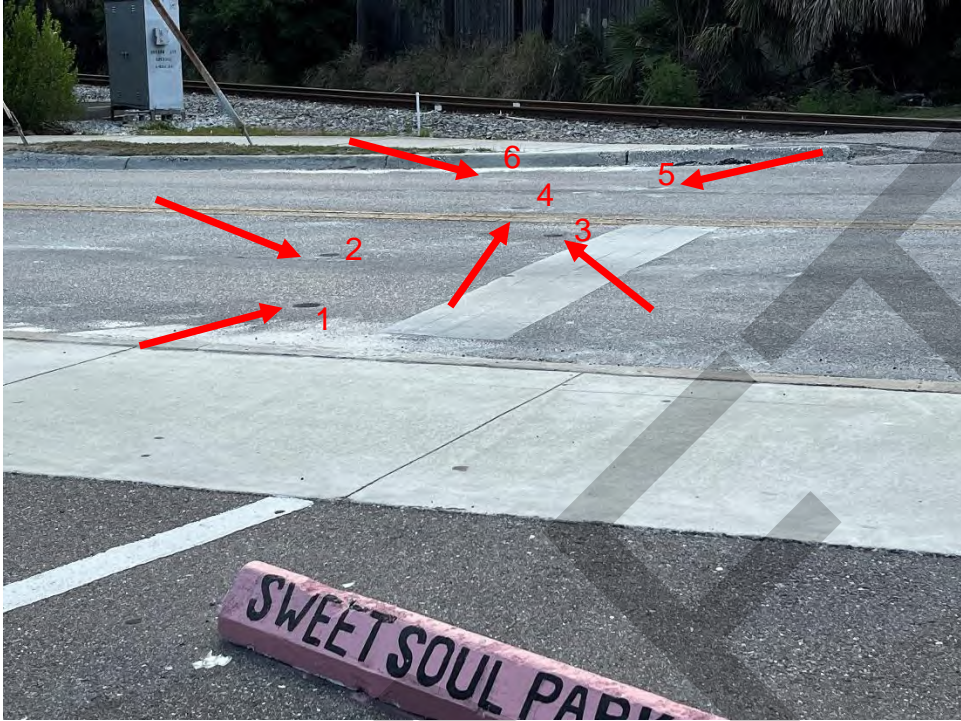
Photograph 1. S. Howard Borehole Locations N of Selmon Expwy, taken from Sweet Soul parking lot
