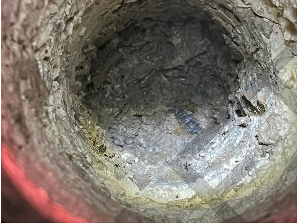
Photograph 3. Rebar within the Borehole #5 on north side (2 feet below asphalt surface)
