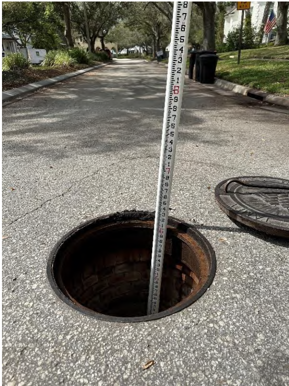
Manhole at the intersection of W Parkland Blvd and S Forest Dr confirms the 90-degree turn of the 48"x76" ERCP
