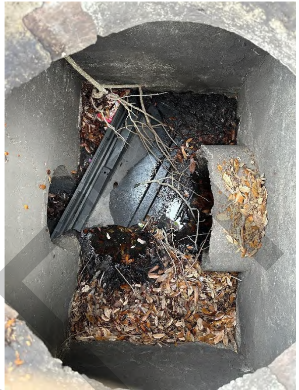
Confirmed inlet on S Moody Ave has an 18" RCP that runs to the west through the school parking lot for St. John the Baptist Greek Orthodox Church
