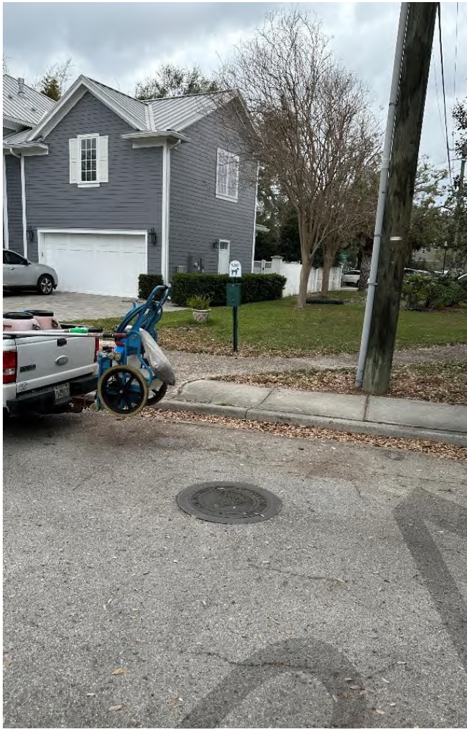
Manhole at the intersection of W Parkland Blvd and S Lakeview Rd. Confirmed a 36" RCP along W Parkland Blvd and a 19"x30" ERCP connecting from S Lakeview Rd
