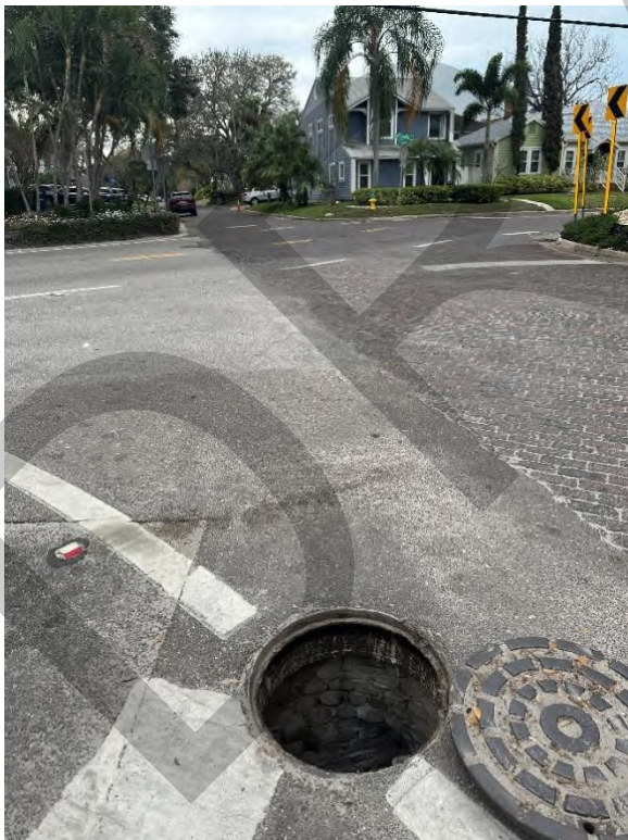
Manhole near the intersection of W Estrella St and S Habana Ave investigated to confirm 60" RCP along S Habana Ave
