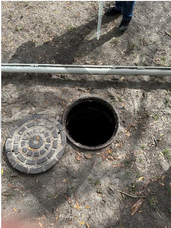
Manhole near the southwest corner of St. John the Baptist Greek Orthodox Church building that connects the 18" RCP from Moody Ave S to the 24" RCP that conveys water north to W Swann Ave
