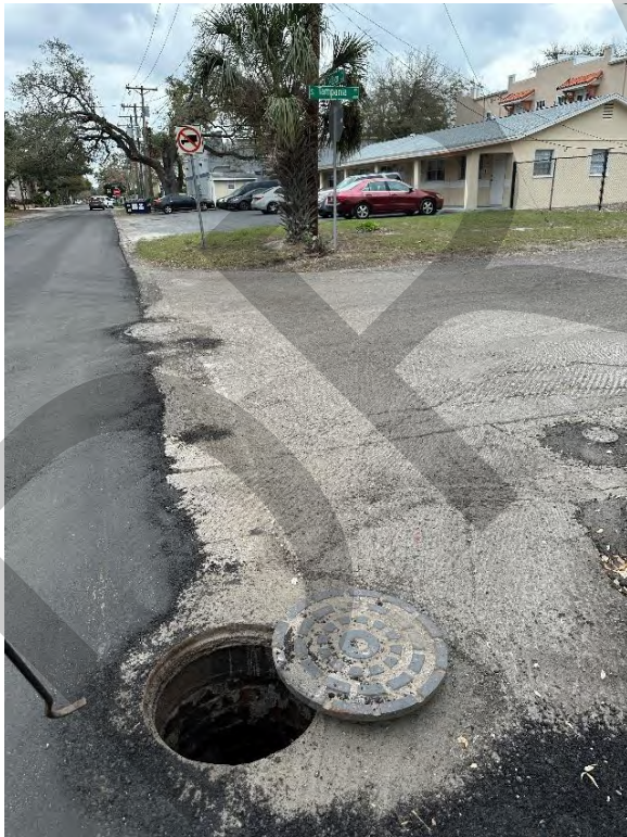
Manhole at the intersection of W De Leon St and S Tampania Ave. Confirmed 18" pipe to the west along W De Leon with a 15" pipe coming in from the north
