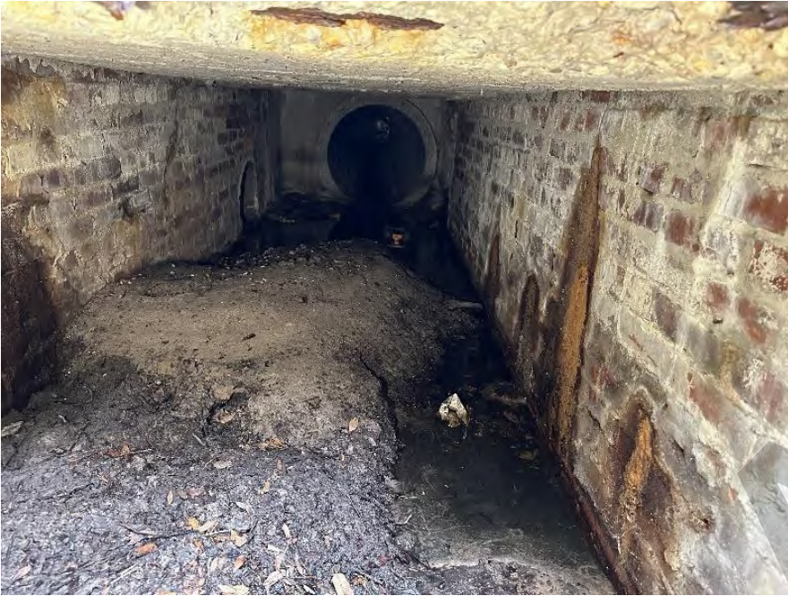
42"x48" Box Culvert bend at the intersection of W De Leon St and S Oregon Ave.
