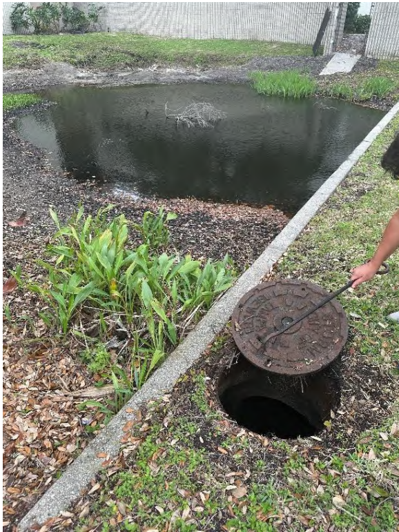
Opened manhole confirms that pipe from W Palm Drive bypasses the stormwater pond adjacent to The Atrium on Bayshore
