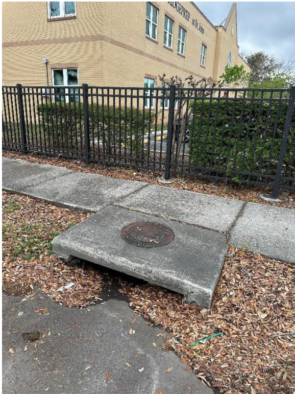
Confirmed inlet on S Moody Ave has an 18" RCP that runs to the west through the school parking lot for St. John the Baptist Greek Orthodox Church
