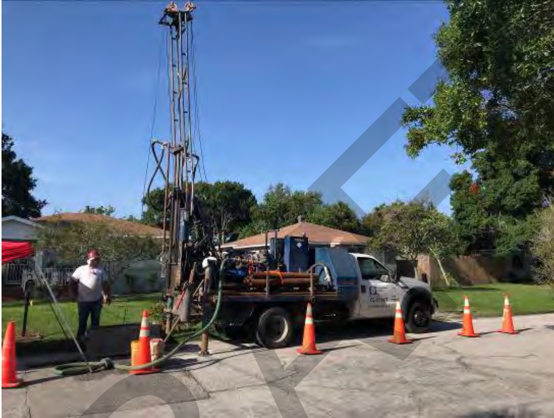
Figure 3: Performing SPT Borings (photographed July 2, 2018)
