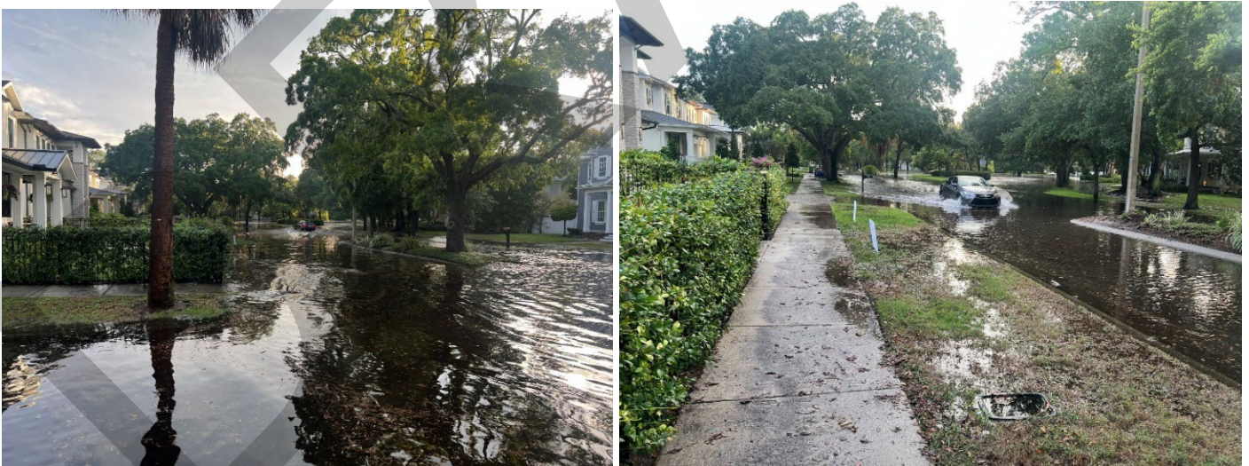
Figure 2-8 – Observed Flooding on June 14, 2024
