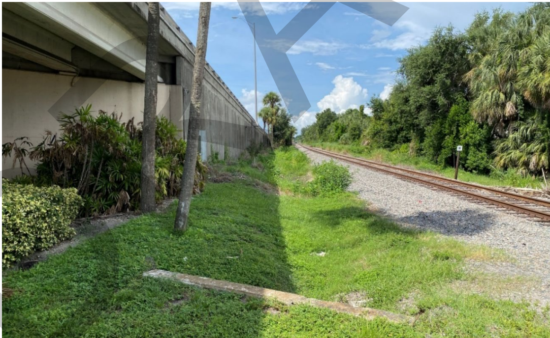
Figure 5-26 – Existing shallow ditch system between Selmon Expressway & CSX Railroad
